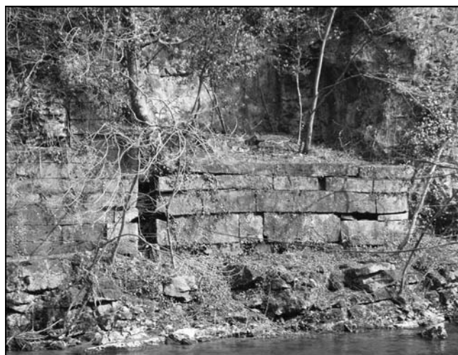
Stone-lined pit that held a water wheel, dating from around 1800, on the High Tor bank of the River Derwent.
